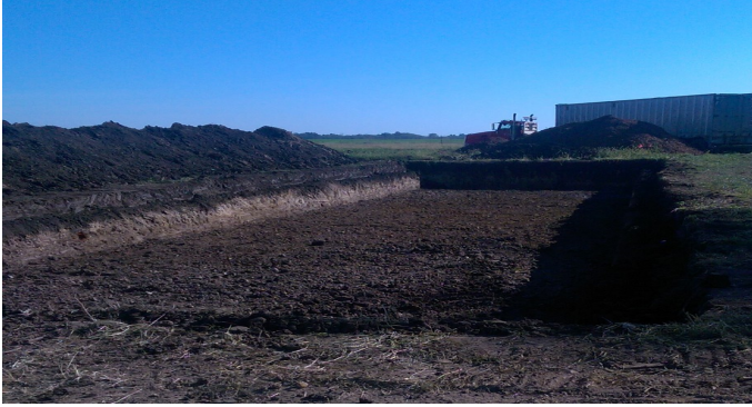
Installing a "Bio-Reactor" for water management
